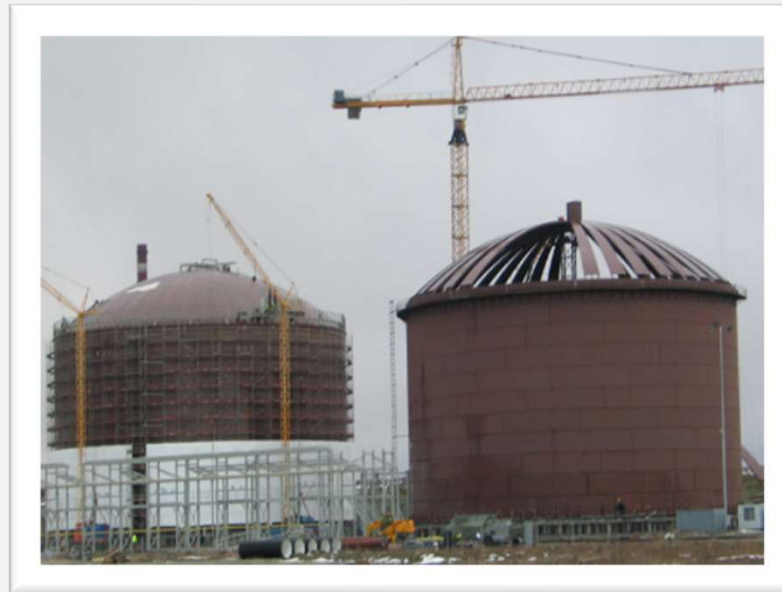
Kohimo project: Estonia, Sillamäe Terminal, 2017-2020 2 x 47 200 m 3 + steel structures + pipelines
